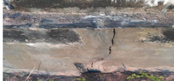
2-rasm. Agressiv muhitdagi poydevorlar holati
